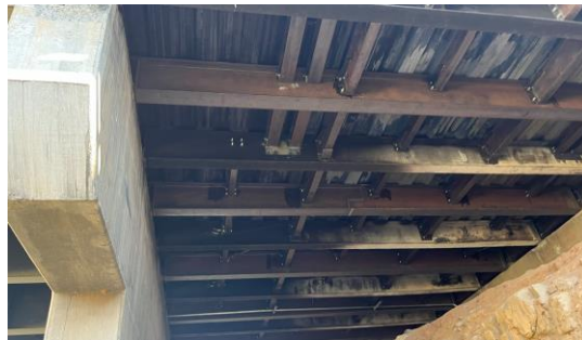
Fig. 5. Installation of New Structural Steel Members
