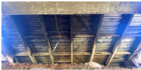
Fig. 1. Underside of Span 1
