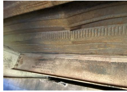
Fig. 4. Separation of Permanent Shutters
