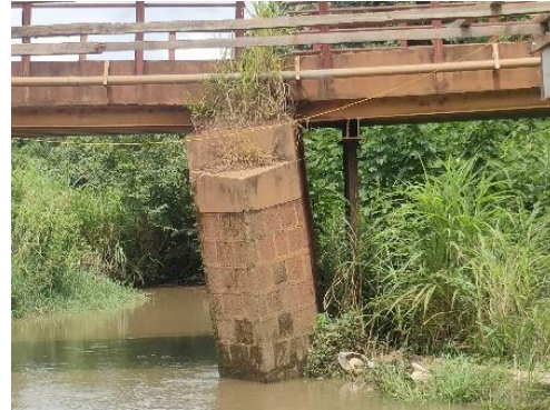
Fig. 2. Bridge N7 View of pier
